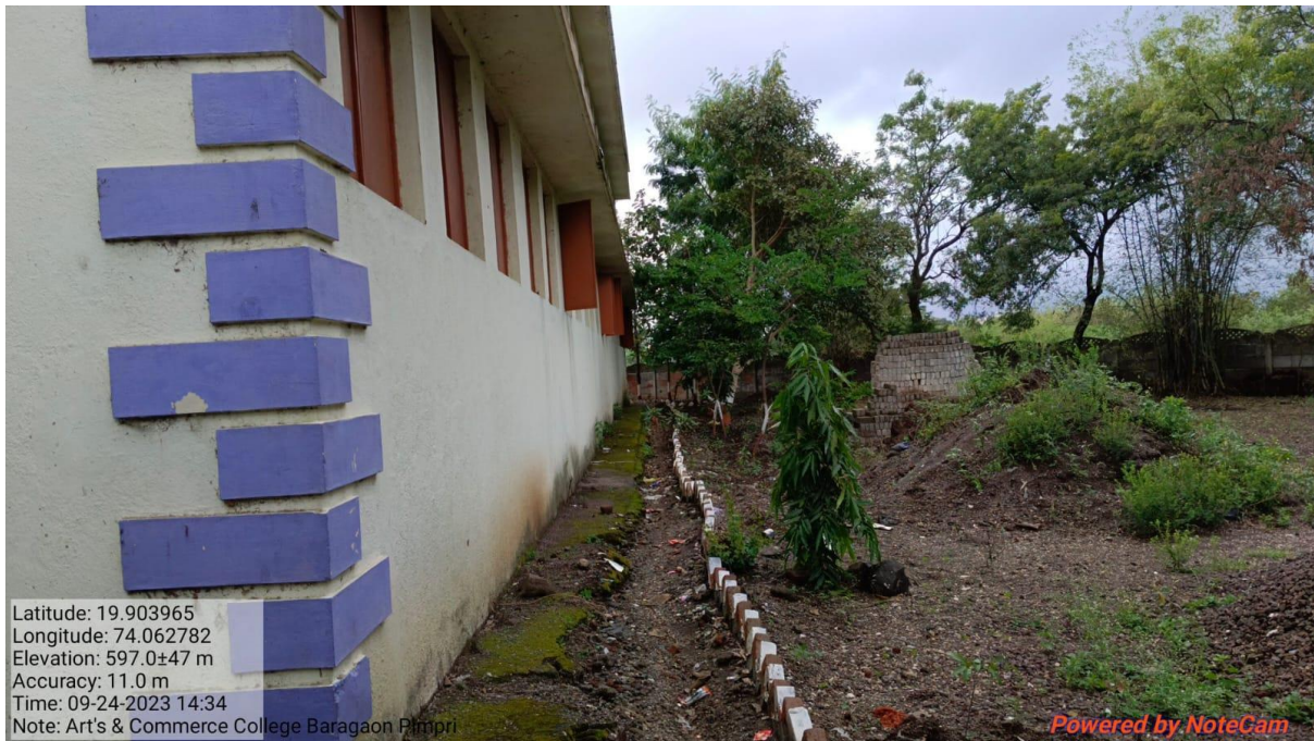
Rain Harvesting in college Campus
